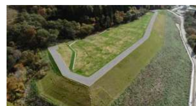
Reinforcement work by soil stabilization at the Yatani Mine Tailings Dam (completion)
