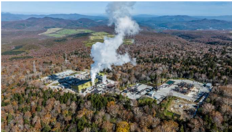
Appi Geothermal Power Plant
