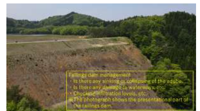
Example of tailings dam management (Osarizawa Mine)
