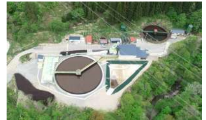
Acid mine drainage treatment facilities (Yatani Mine)
