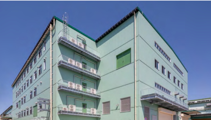
Rolled Product Line No. 3, Sambo Plant
