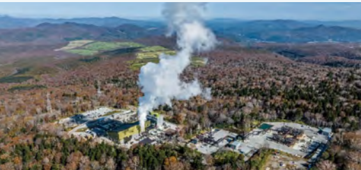
Appi Geothermal Power Plant
