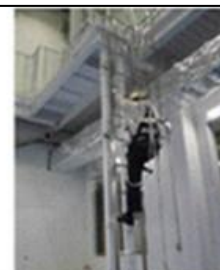
Exterior Ladder &amp; Safety Blocks
