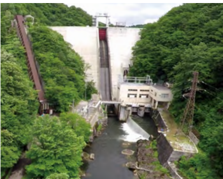
Komatagawa Power Plant No. 4
