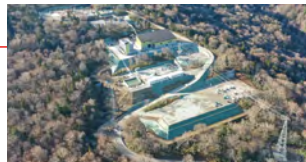
Appli Geothermal Power Plant (entire construction area)
