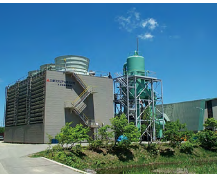
Onuma Geothermal Power Station
