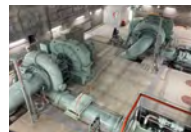
Inside of the Komatagawa New Power Plant (water turbines and generators)
