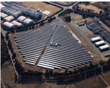
Makabe Solar Power Plant
