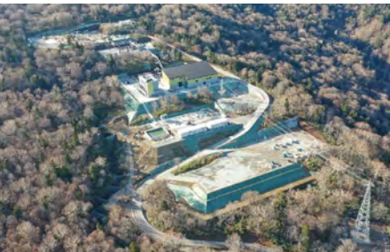
Construction at the Appi Geothermal Power Plant
