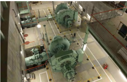
Water turbine generators at the Komatagawa New Power Plant
