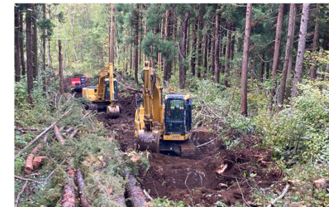
Work road construction and root removal (October 2022)
