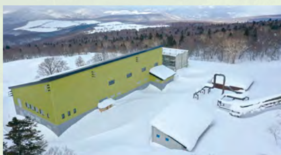
Appi Geothermal Power Plant building
