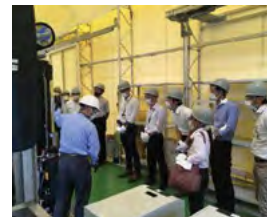
Viewing CO 2 separation and recovery equipment
