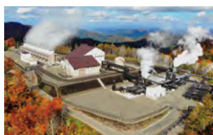
Wasabizawa Geothermal Power Plant
