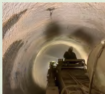
Spraying at section 2 of Komatagawa New Power Plant
