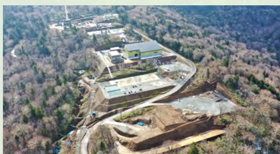
Appi Geothermal Power Plant (under construction)
