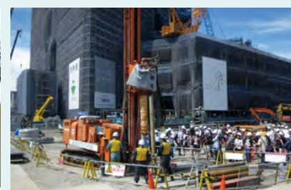
Construction of a practical geothermal heat pump system (Tokyo Skytree)
