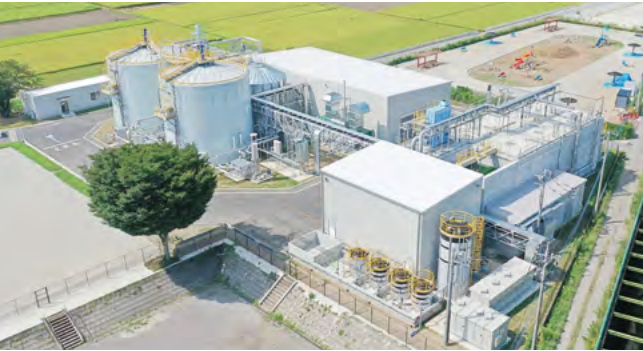
Food waste biogasification The Company promotes a recycling business that performs biogasification (methane fermentation) on the food waste output from locations such as food service industries, retail stores and factories to generate renewable energy (electricity), and thereby achieve both the suitable treatment of waste and the supply of energy to society.
