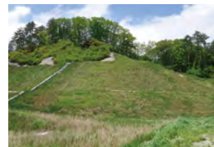
[Rainfall infiltration control and reforestation] Contamination containment work by slope seeding with Chipcrete at the Komagi Mine
