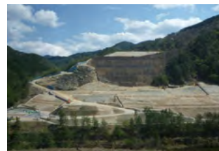
[Earthquake countermeasures] Reinforcement work by soil stabilization at the Ikuno Mine Tailings Dam
