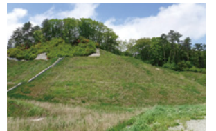
Contamination containment work by slope seeding called Chip-crete at the Komagi Mine
