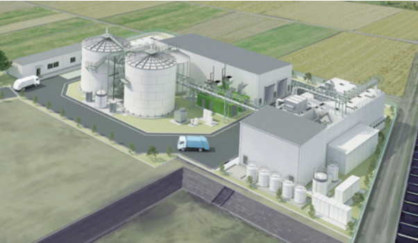
Food waste biogasification (New Energy Fujimino Co., Ltd.: Scheduled to start operation in September 2020) The Company promotes a recycling business that performs biogasification (methane fermentation) on the food waste output from locations such as food factories and retail stores to generate renewable energy (electricity), and thereby achieve both the suitable treatment of waste and the supply of energy to society.
