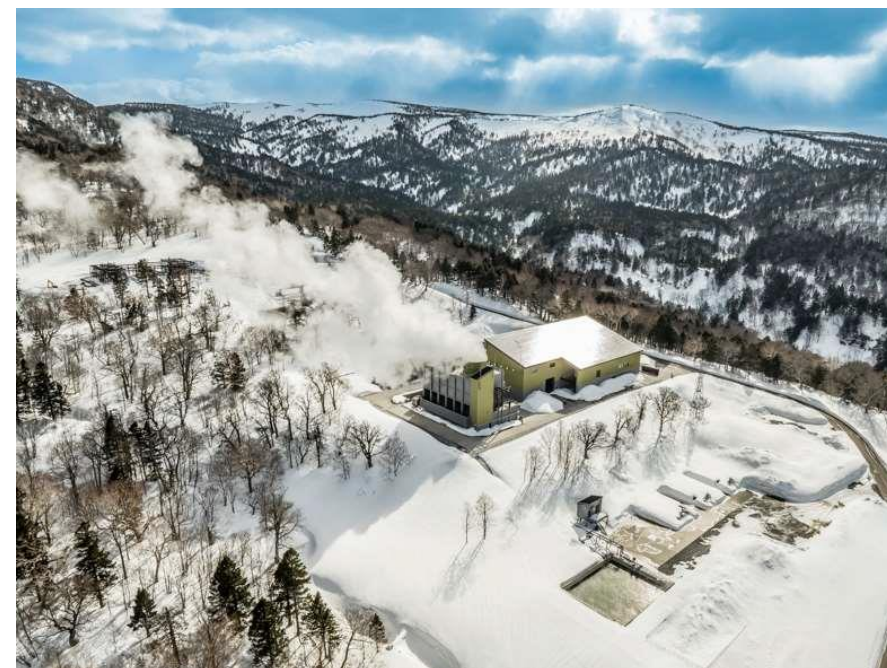
Appi Geothermal Power Plant in Winter
