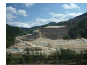
Reinforcement work by soil stabilization at the Ikuno Mine Tailings Dam
