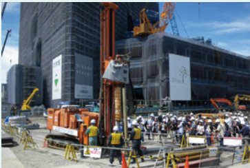
Construction of a practical geothermal heat pump system (Tokyo Skytree)
