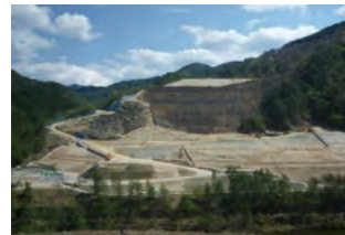
[Earthquake countermeasures] Reinforcement work by soil stabilization at the Ikuno Mine Tailings Dam
