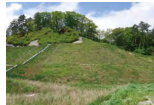
[Rainfall infiltration control and reforestation] Contamination containment work by slope seeding with Chipcrete at the Komagi Mine
