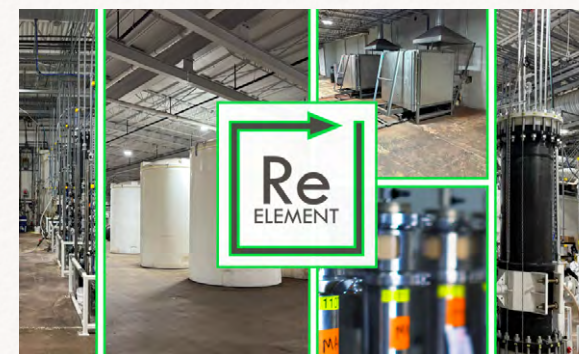
Large-scale commercial plant scheduled to begin operations in 2026: Marion Advanced Technology Center
