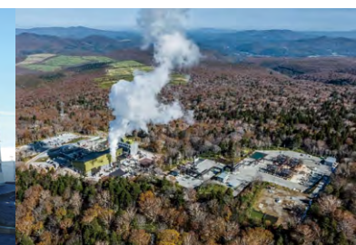
Appi Geothermal Power Plant
