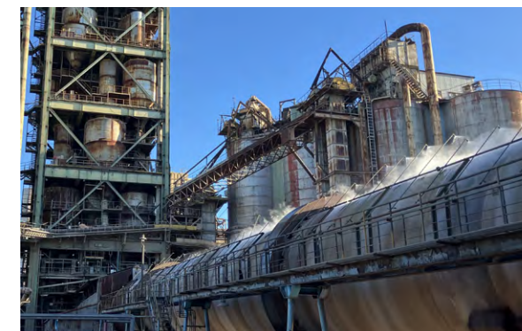
MUCC Kyushu Plant Kurosaki District (cement kiln and preheater)
