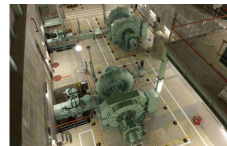
Komatsugawa New Power Plant (water turbine generator)
