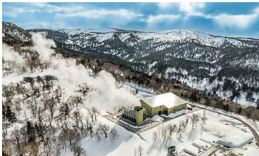
Appi Geothermal Power Plant in winter
