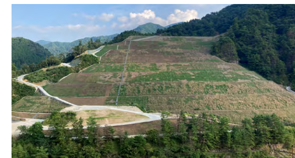
Kyuhodani tailings dam (Ikuno Mine)
