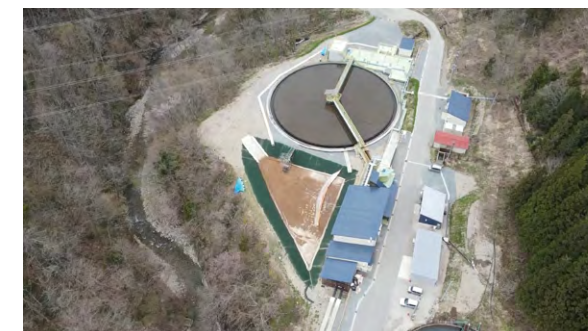
Acid mine drainage treatment (Yatani Mine)
